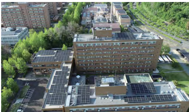
Installation of solar energy power generation facilities (Higashi-Hiroshima Campus)
